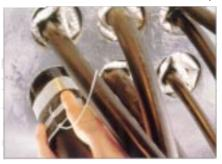
With the sealant strips lubricated, the product is simply wrapped around the cable and easily slides into the duct. The bladder is then inflated with a gas pressure tool which presses the sealant coating against the duct wall and the cable. Upon removal of the filling tube,
