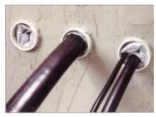
an automatic gel valve system reliably retains the gas pressure in the Rayflate duct seal.
