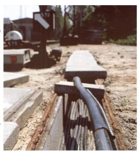
1 CRSM wraparounds are used in a railway goods yard in Germany to restore the insulating, sealing and mechanical protection functions of damaged cable oversheaths.
